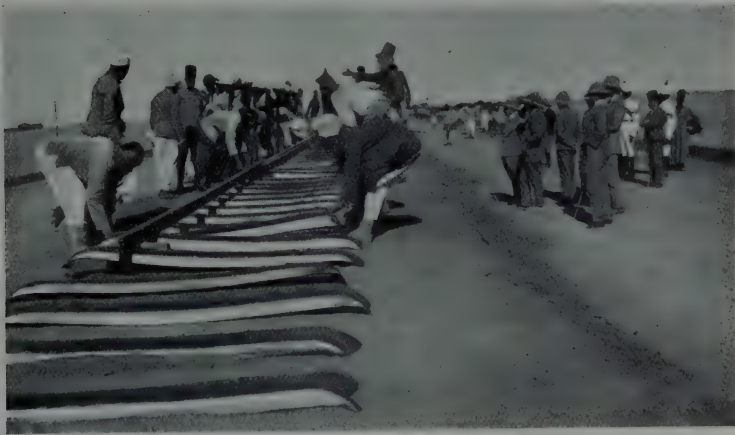
LAYING THE ATBARA-RED SEA RAILWAY.
